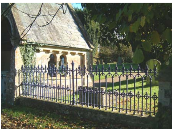
St Nicholas Church. A slate roof on the lych gate limestone walls and fine quality iron railings .
